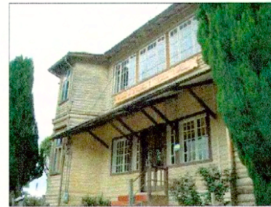
Vista parcial fachada principal
