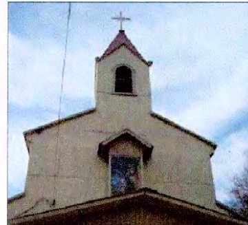
Detalle fachada principal
