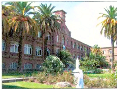
Vista fachada principal
